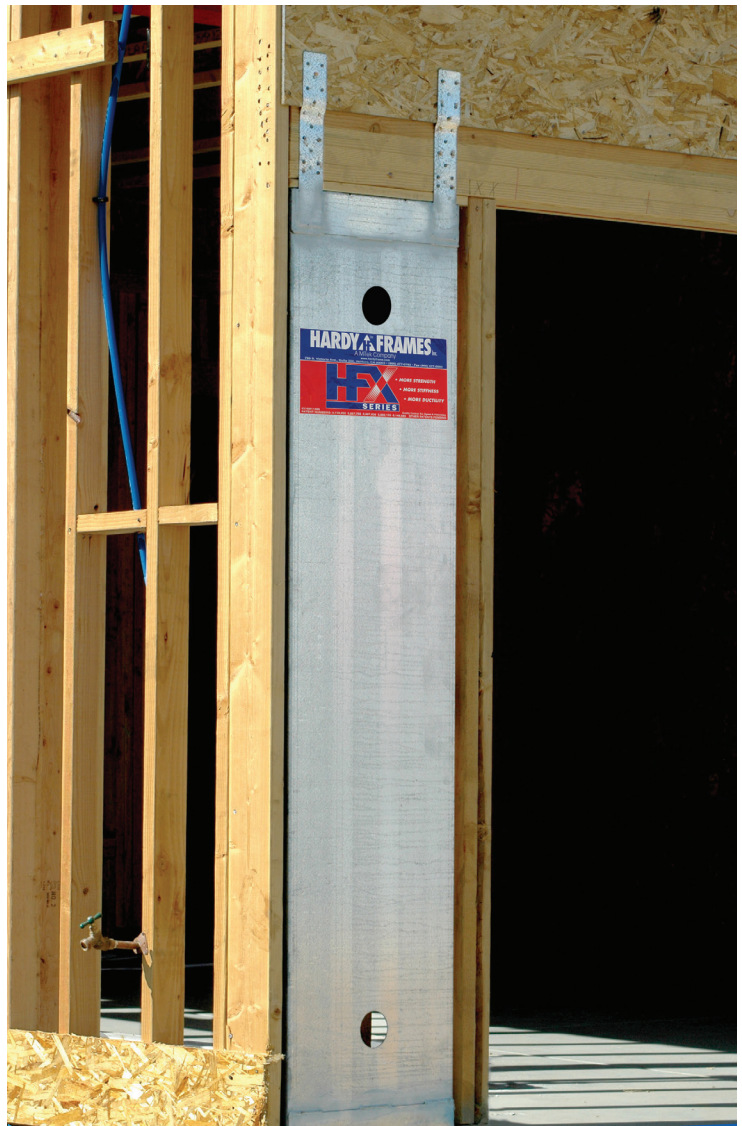
GARAGE FRONT WITH STRAPS
