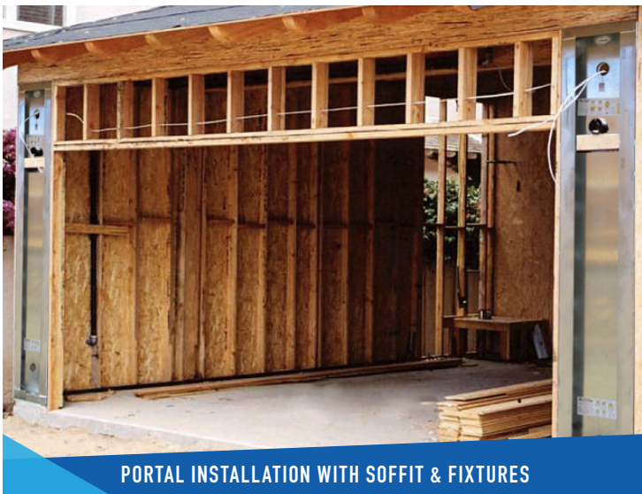
GARAGE FRONT HANGING SOFFIT
