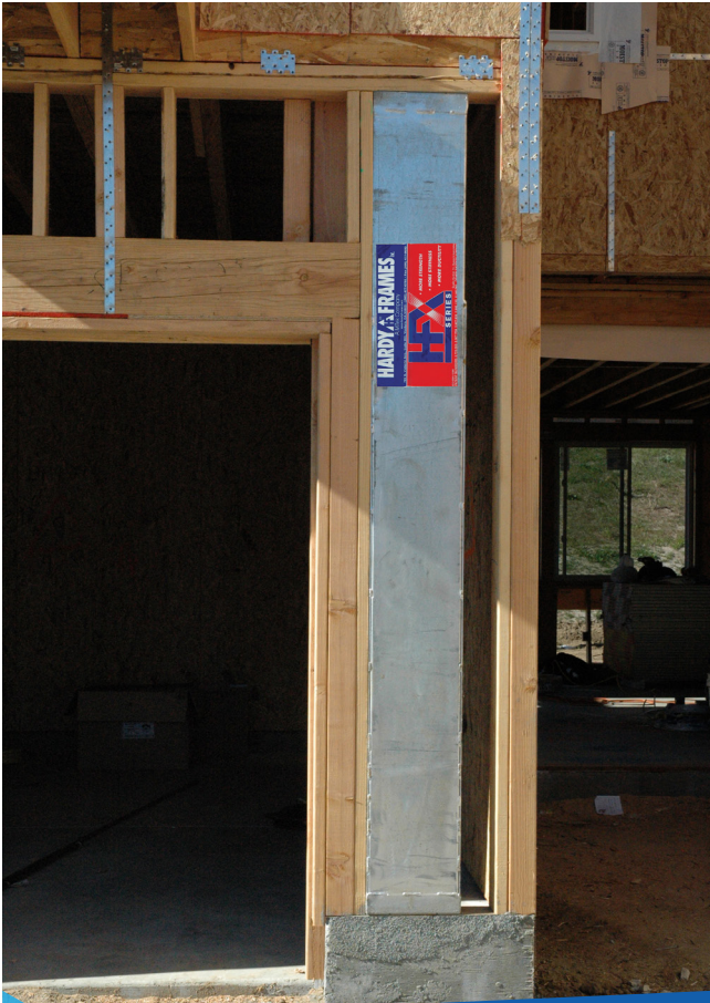
GARAGE FRONT TOP PLATE CONNECTION
