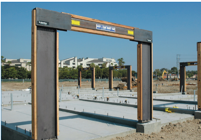
SPECIAL MOMENT FRAMES NEW CONSTRUCTION
