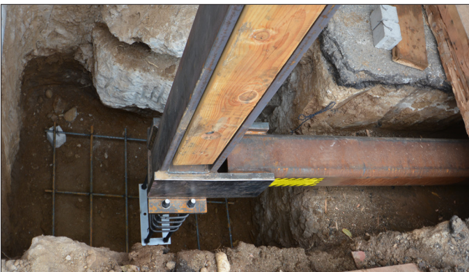
HARDY FRAME PICTURE FRAME INSTALLATION
