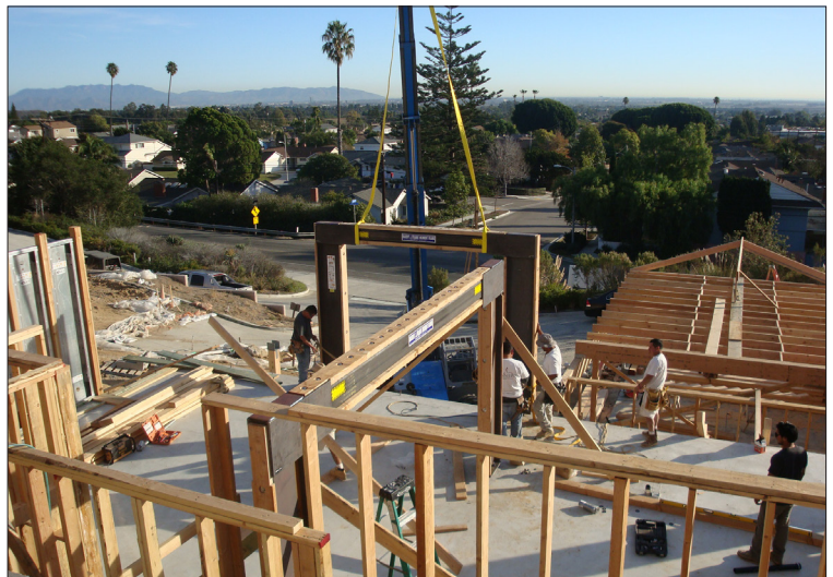
SPECIAL MOMENT FRAMES IN NEW CONSTRUCTION
