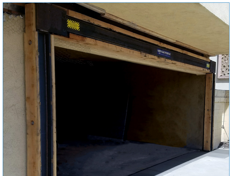
SPECIAL MOMENT FRAME IN RETROFIT APPLICATIONS
