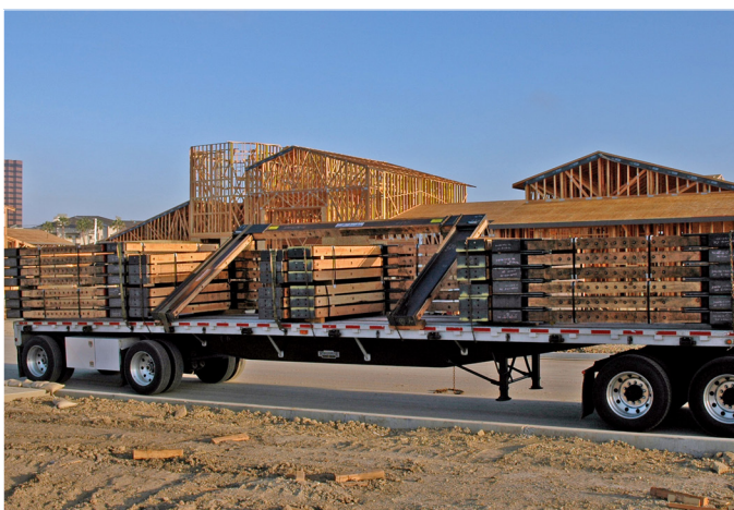
SPECIAL MOMENT FRAMES DELIVERY TO JOB SITE
