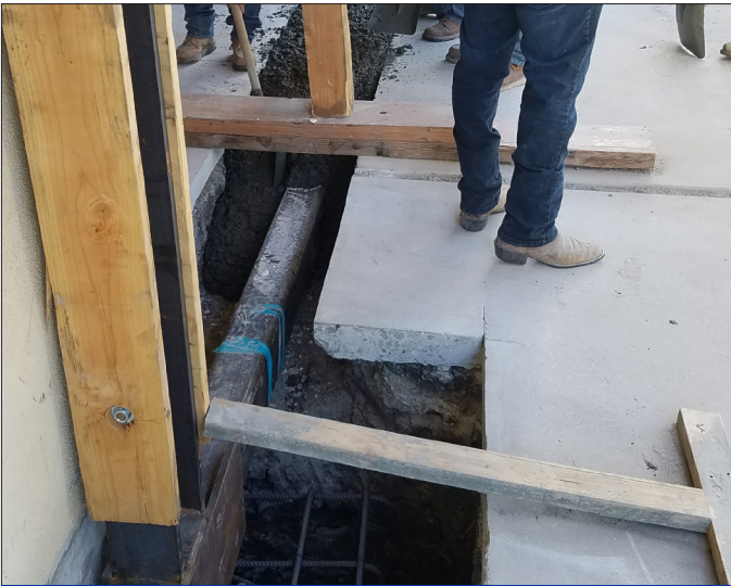
INSTALLING HARDY FRAME PICTURE FRAME
