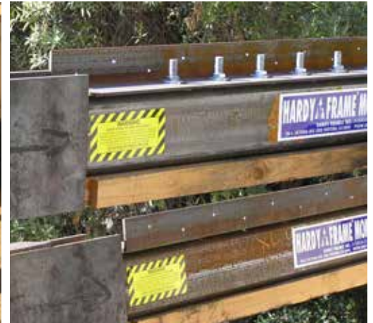
ANGLES FOR SHEAR TRANSFER
