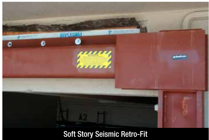
Standard SidePlate® connection
