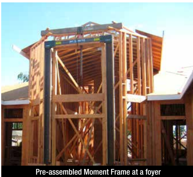
Pre-assembled 2-story Hardy Frame Moment Frames
