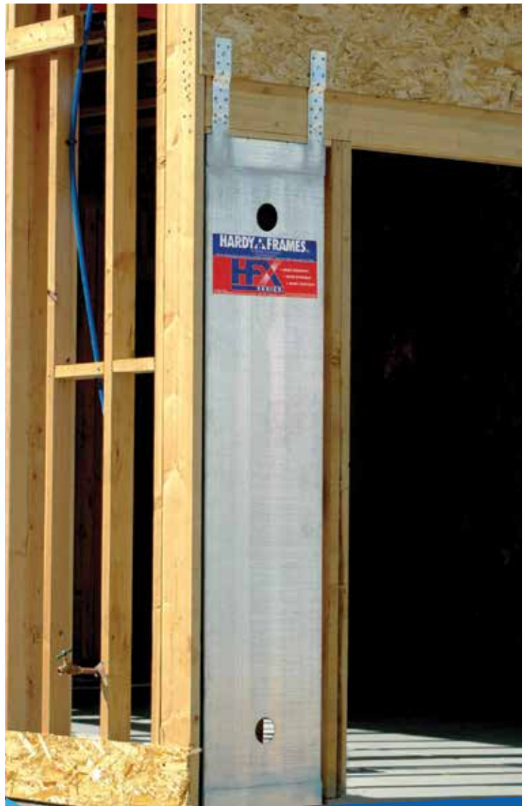
GARAGE FRONT WITH STRAPS
