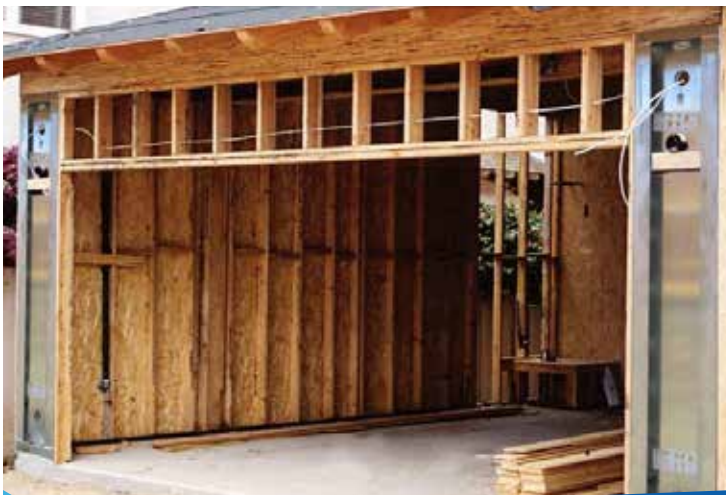
PORTAL INSTALLATION WITH SOFFIT & FIXTURES
