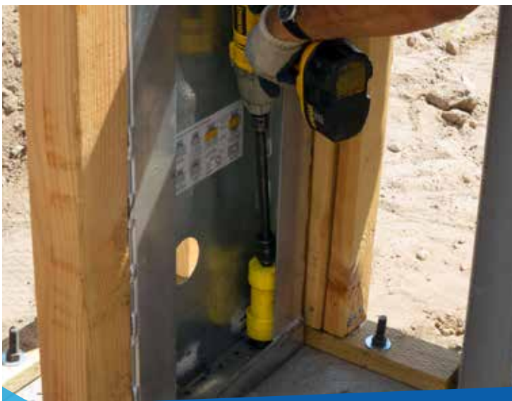
BOTTOM CONNECTION WITH DEEP SOCKET & SWIVEL
