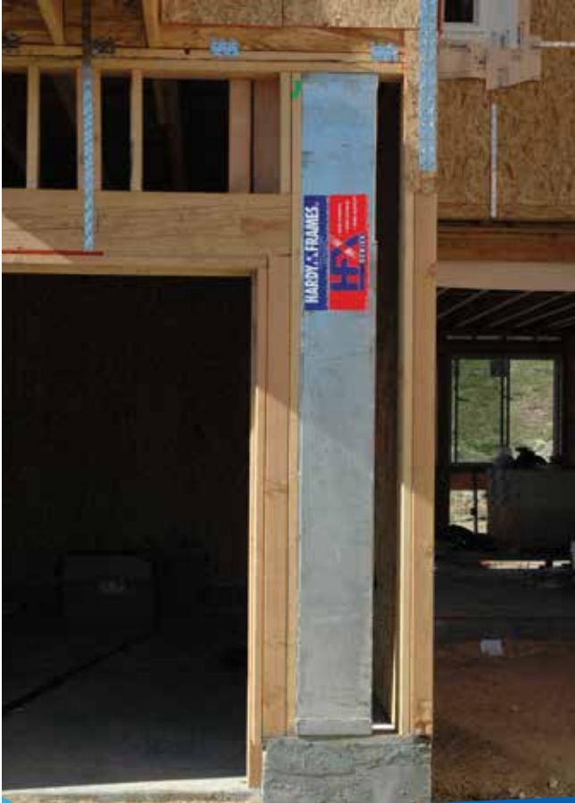
GARAGE FRONT TOP PLATE CONNECTION
