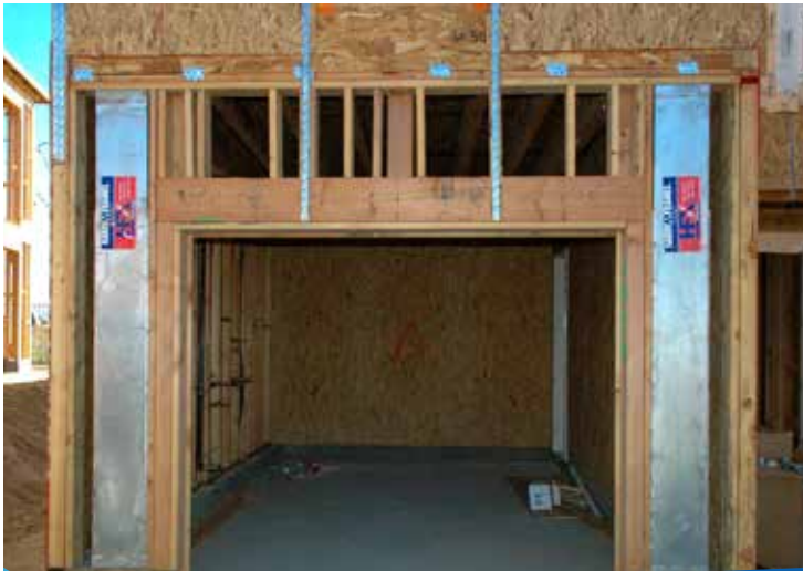
GARAGE FRONT HANGING SOFFIT
