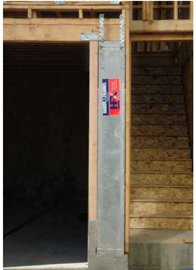
GARAGE FRONT WITH STRAPS
